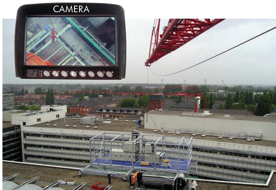
*Spierings cranes are equipped with a zoom-camera on the trolley ensuring high precision. The operator keeps perfect overview at all times and never works blindly. The cabin's high position ensures excellent overview which makes operation safer.*
